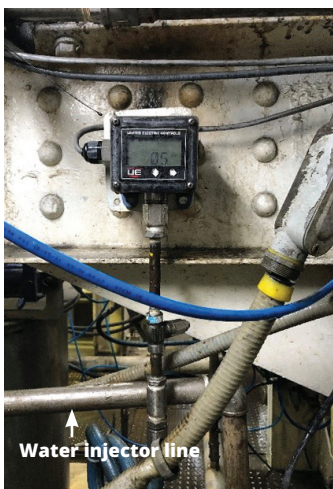
Excelsa installed on a water injector line of a centrifuge
