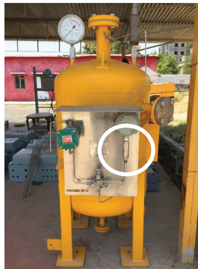
Compact 12 series fitted on extinguishing agent tank
