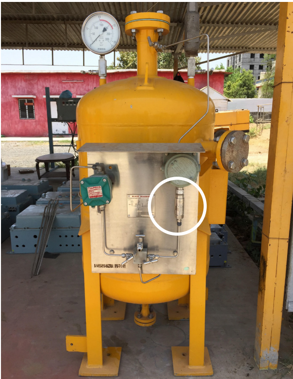
Figure 4. Actual tank in a RSFPS with 12 series instrument circled.
