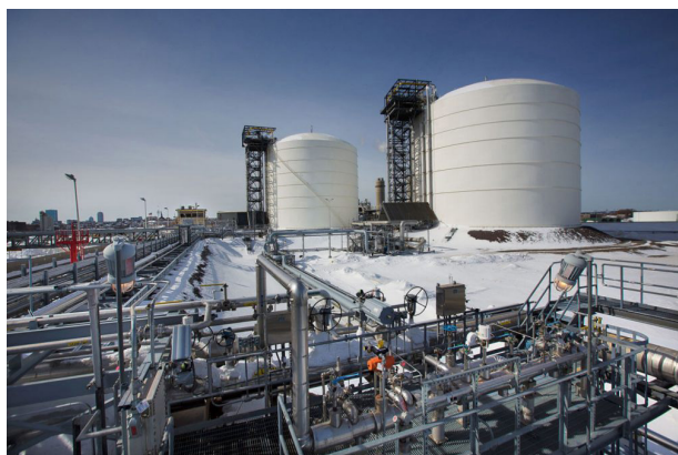
Figure 1. An LNG facility during the winter season, with snow build-up.
