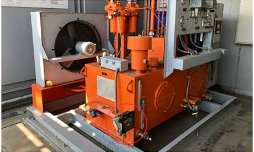
IMAGE 3: Temperature switch used on lubrication system
