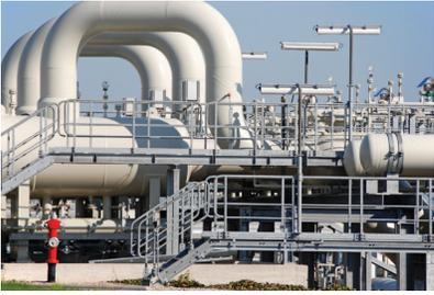
The storage of natural gas is a process whereby gas is injected into the porous rock of depleted reservoirs. In the gas supply chain, storage is particularly important because it compensates for the differences between supply and demand for gas and ensures continuity of supply. Once the gas has been injected it can be withdrawn, depending on demand, and used to ensure a sufficient supply of natural gas to industries and for heating in winter.
